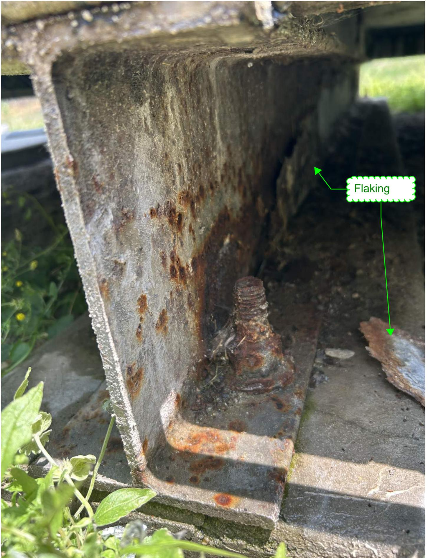
Steel supporting the cooling tower severely deteriorated and must be replaced.
